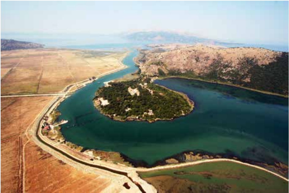
Figure 1. View of Butrint and the Straits of Corfù
