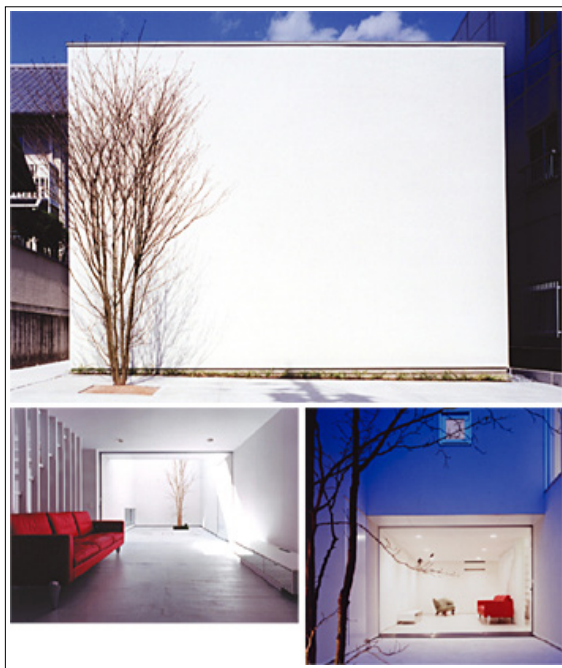
Figure 42 (Top). “House in Minami Danbara”, Hiroshima. Architect: Yamashita Hiroyuki, 2012
