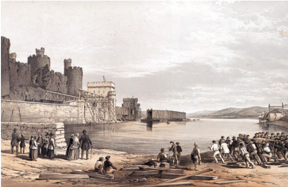
Figure 15 George Hawkins, Lithograph showing the second wrought-iron box girder tube of Robert Stephenson's tubular railway bridge at Conwy being floated into position (September 1848), 300 × 465 mm (image), 370 × 547 mm (paper). Impression digitized by National Library of Wales. © Wikimedia Commons
