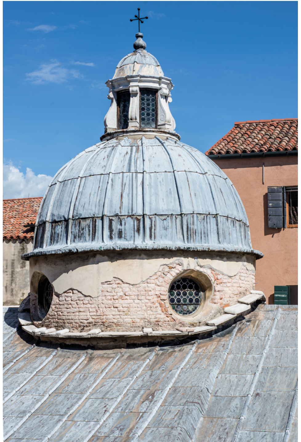
Figure 11 Church of San Giacomo di Rialto, Venice, view of the external dome. Photo © Böhm
