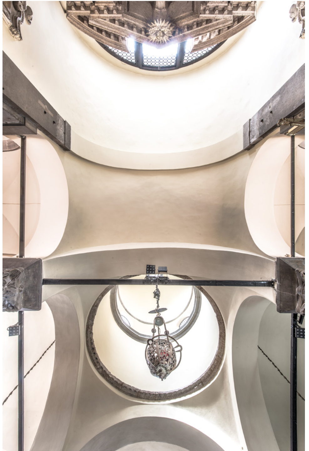
Figure 8 Church of San Giacomo di Rialto, Venice, view of the inner vaults. Photo © Böhm
