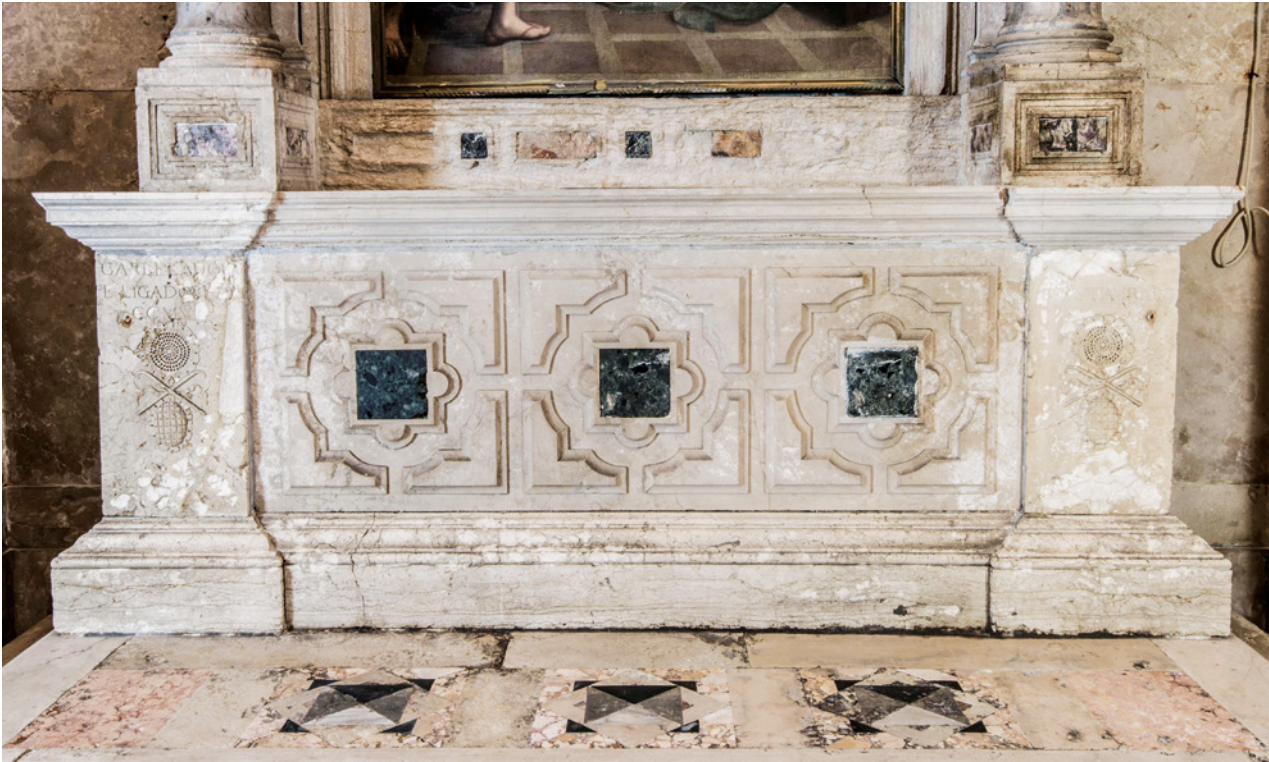
Figure 10 Church of San Giacomo di Rialto, Venice. “Dell’Annunziata” Altar, antependium. Photo © Böhlm
