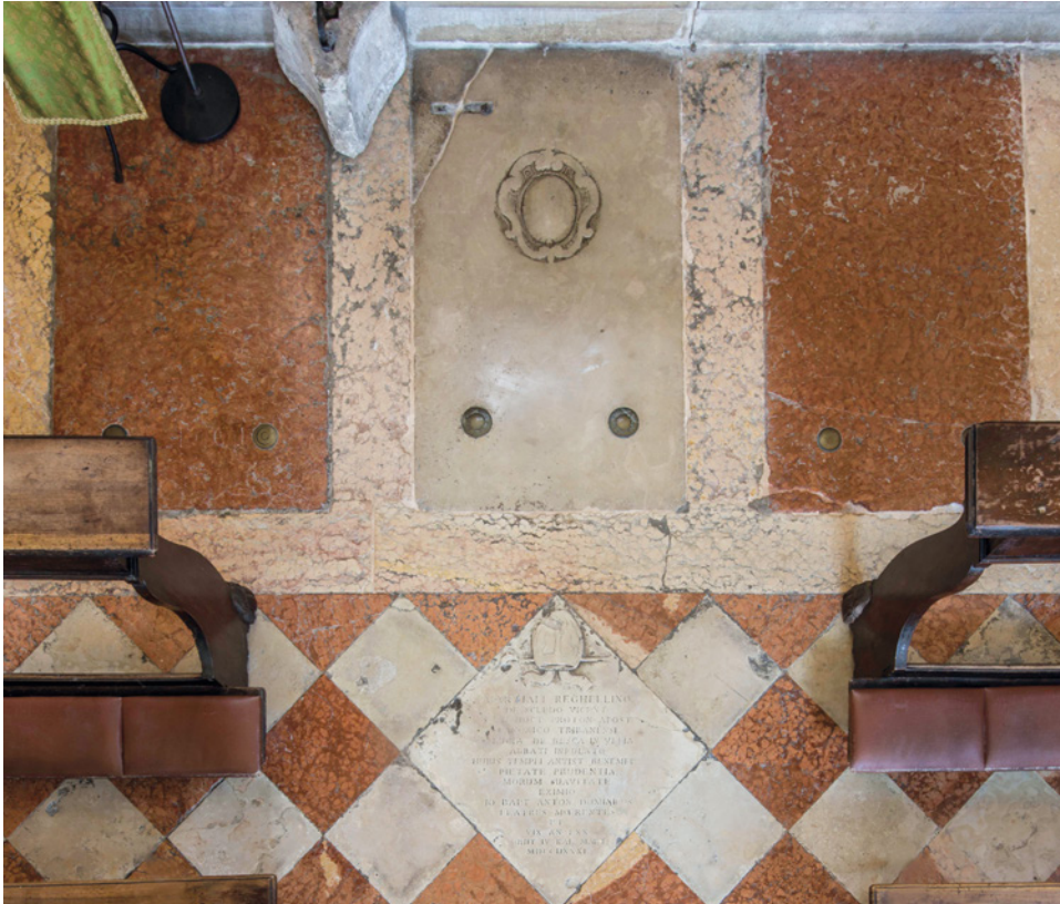
Figure 1 Church of San Giacomo di Rialto, Venice. Pavement with a chequerboard pattern consists of squares of white Istrian stone and red Verona broccade. Photo © Böhm
