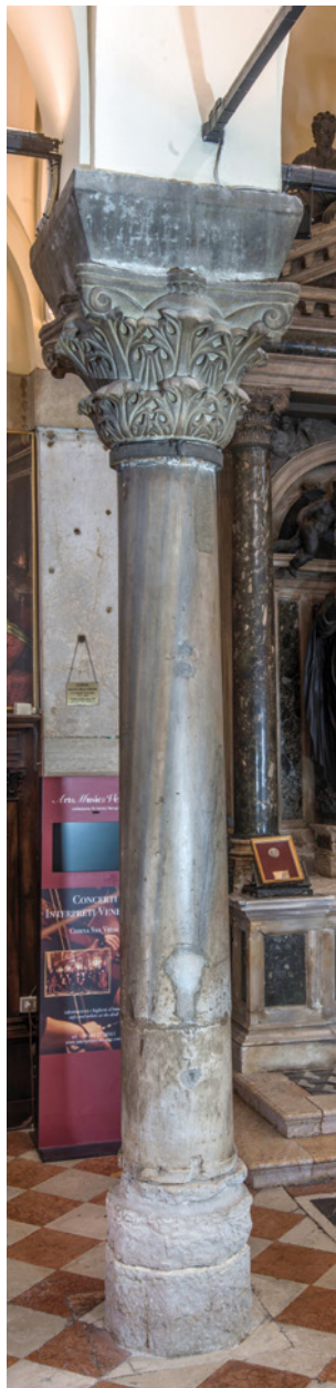
Figure 26 Venice, Rialto, Church of San Giacomo. One of the column made of Proconnesian marble positioned on its base and surmounted by a medieval capital. Photo © Böhm
