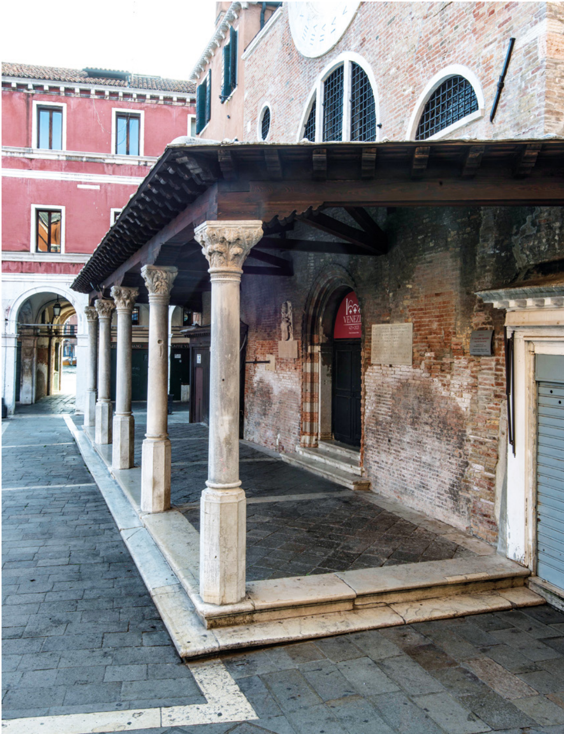
Figure 13 Venice, Rialto, Church of San Giacomo. Lateral view of the portico. Photo © Böhm
