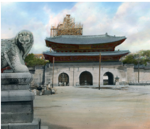
Figure 5 Burton Holmes, Government General Building under Construction . Early 1920s. Hand-coloured lantern slide, 3.5 × 4 inches (8.3 × 10 cm). Courtesy of the Burton Holmes Collection, Department of Art History, University of California, Los Angeles
