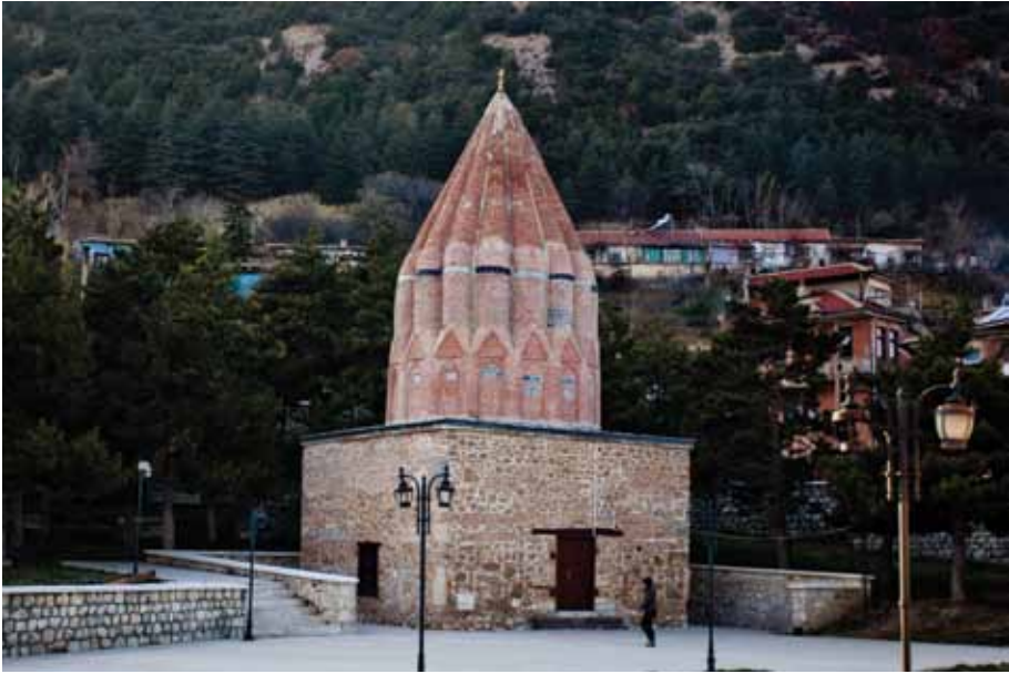
Fig. 13. Akşehir, türbe of Seyyid Mahmud Hayrani, 1224
