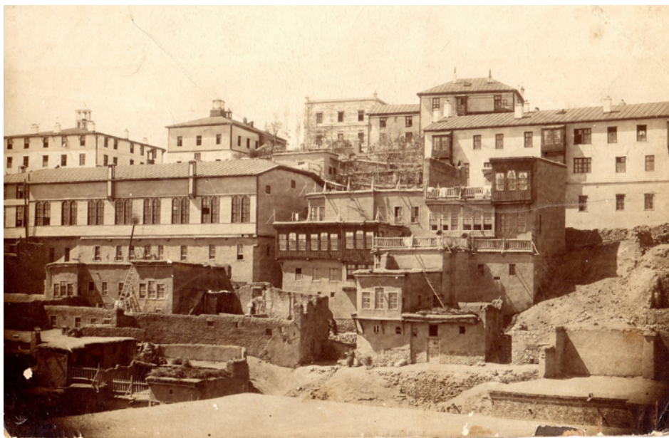
Figure 5. Harput. A view of the town. The Euphrates College buildings can be seen in upper part. Hourig Zakarian collection. Courtesy of Houshamadyan website
