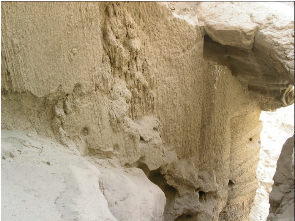
Figure 12. The left wall of stairway Cave 113. The steps have been almost completely eliminated by the water gushing through, with few traces remaining in the lower section of the wall. Notice the space appositively carved in the reveal for the open shutter, aiming at allowing for the maximum width of the passage
