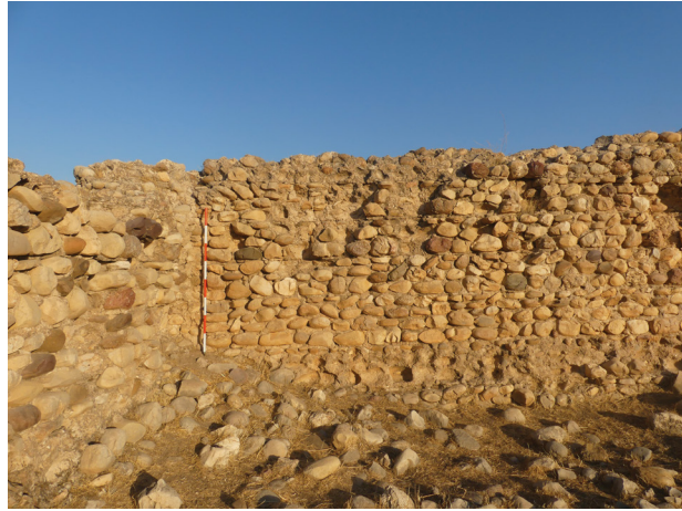
Figure 10 Characteristics of stone placement in the horizontal banks (western internal wall)
