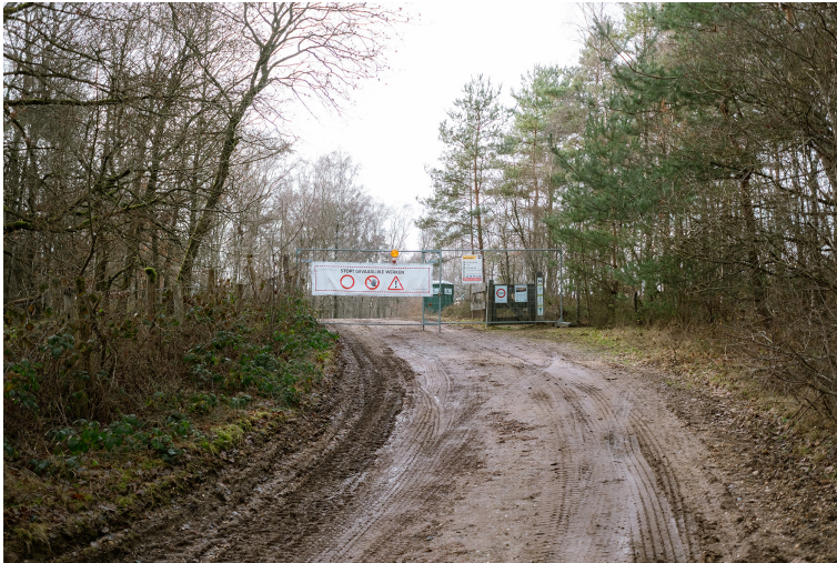
Figure 14 Former entrance to the site, currently blocked due to the restoration works. 2026. Maasmechelen, Belgium. © Kseniia Obukhova
