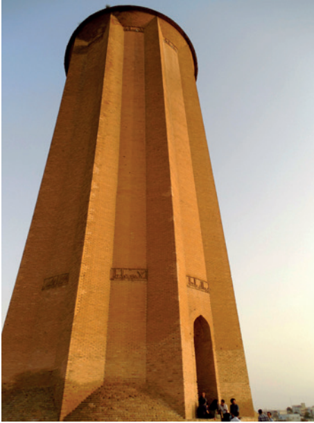
Figure 2. View of the Gonbad-e Kāvus tower from south
