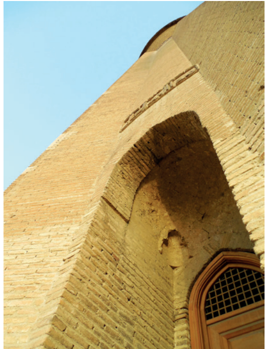
Figure 6. Arched entrance of the tower of Gonbad-e Kāvus with one of the two stucco niches
