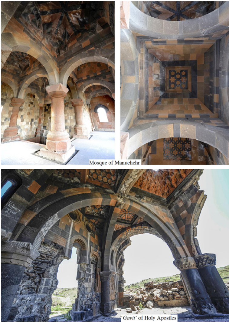
Figure 18 Ceilings, vaults and capitals of columns in Manuchehr mosque and the Holy Apostles 'gavit', Ani, both c. 1200. © H.H. Khatcherian
