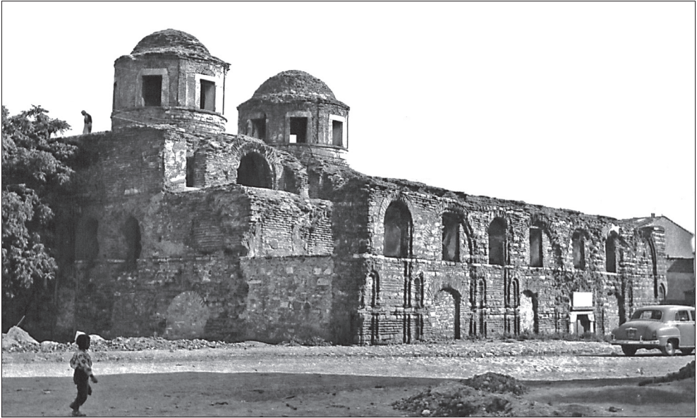
Figure 4 Cahide Tamer, photo of the Church of Monastery of Lips (present-day Fenari İsa Mosque). 1959. © Cahide Tamer Historic Buildings Restoration Projects Collection, Suna Kıraç Library, Koç University, Istanbul, Turkey
