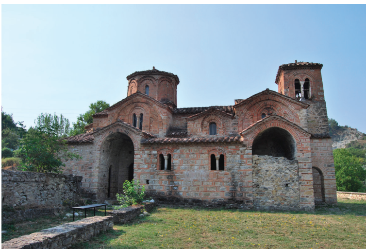
Figure 1 Church of Saint George (North view). 11th-13th cc. Brickwork. Omorfokklisia, Kastoria, Greece. © Elena De Zordi
