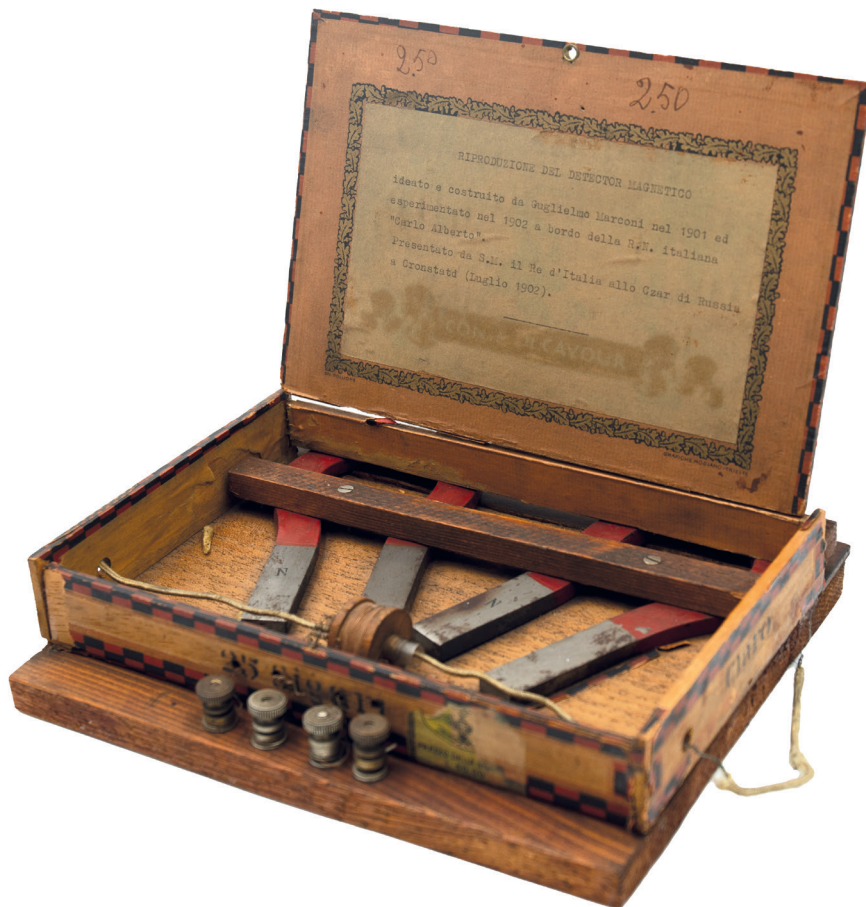
Reproduction of the magnetic detector in a cigar box. 1930s. Inv. IGB-2139
