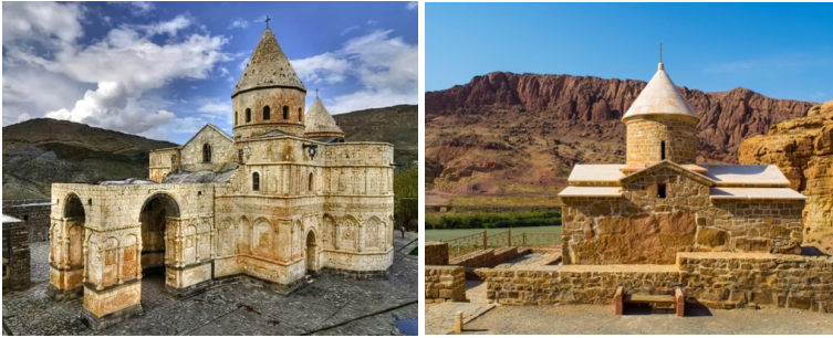
Figure 10 S. Thaddaeus Monastery © Marouti A. and Dzor Dzor Chapel after restorations © Wiki Commons. The chapel was dismantled and moved 600 meters following the construction of a dam
