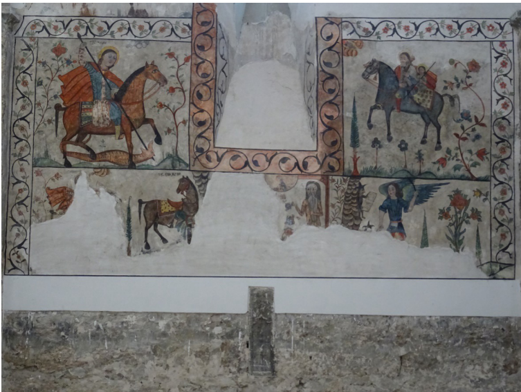
Figure 13 Haftvan, S. Gevorg: mural paintings recently discovered and restored (details). 2018. © Boriani M.
