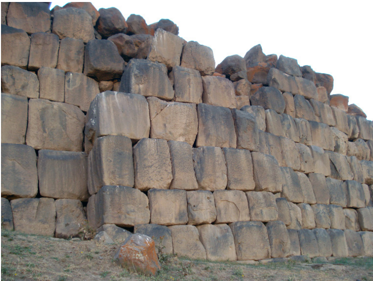
Figure 11 Detailed view of one of the buttresses. Note the lifting tenon on the left side of the buttress
