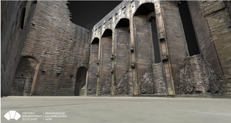
Figure 4 A photorealistic 3D model of Linlithgow Palace Chapel, created by combining the accurate geometry of the laser scan, and the colour imagery from the photographs, Historic Environment Scotland
